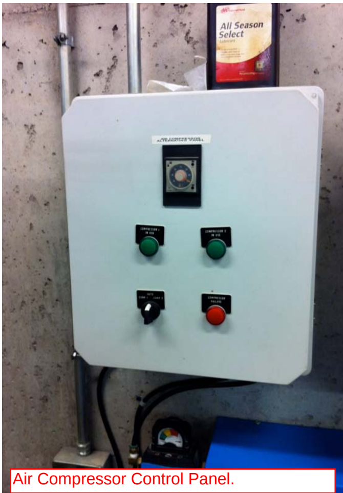
Air compressors for pneumatic controls.
