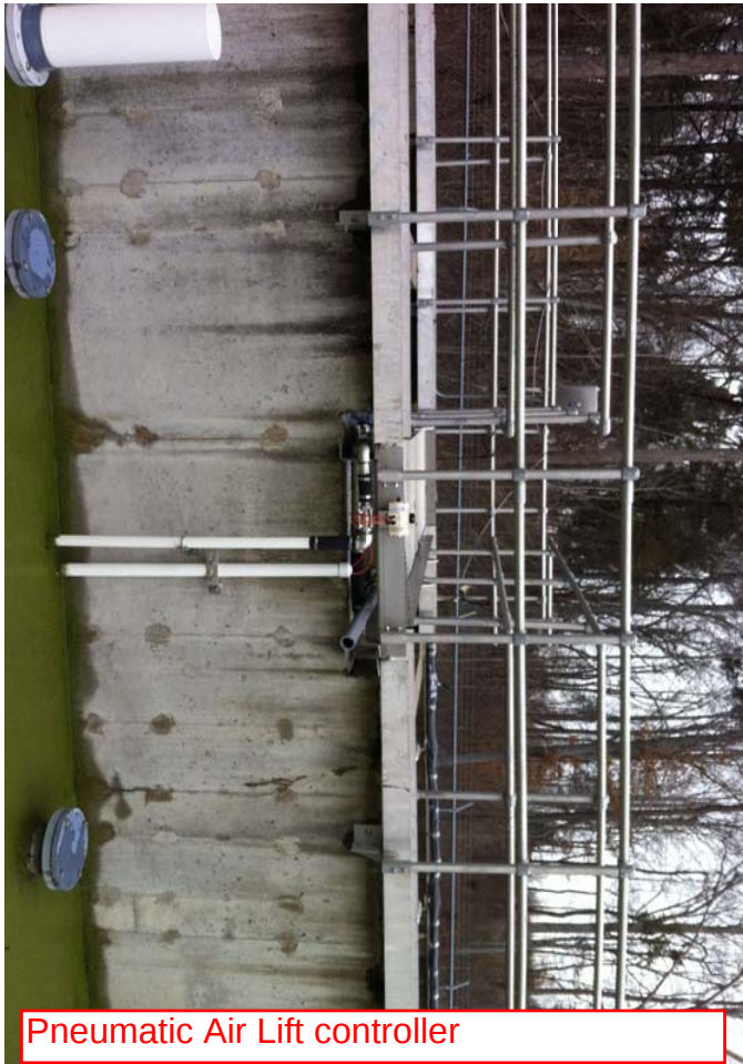
Second stage aeration tank (out of service).
