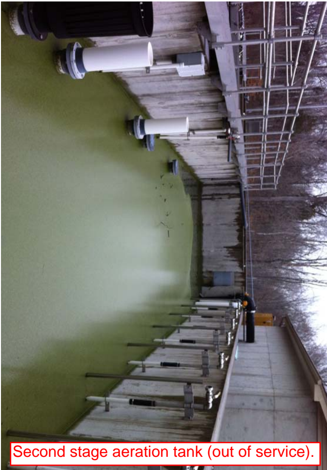
PVC air pipes that have been replaced.
